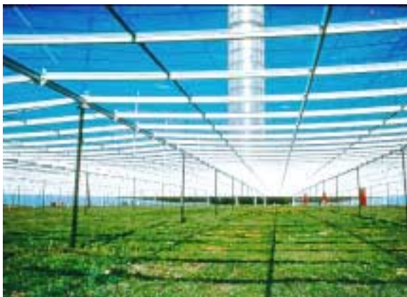
Fig. 6. Glass roof of the prototype plant at Manzanares, Spain. It resisted heavy storms for many years without harm and proved to self-cleaning thanks to the occasional rain showers.
