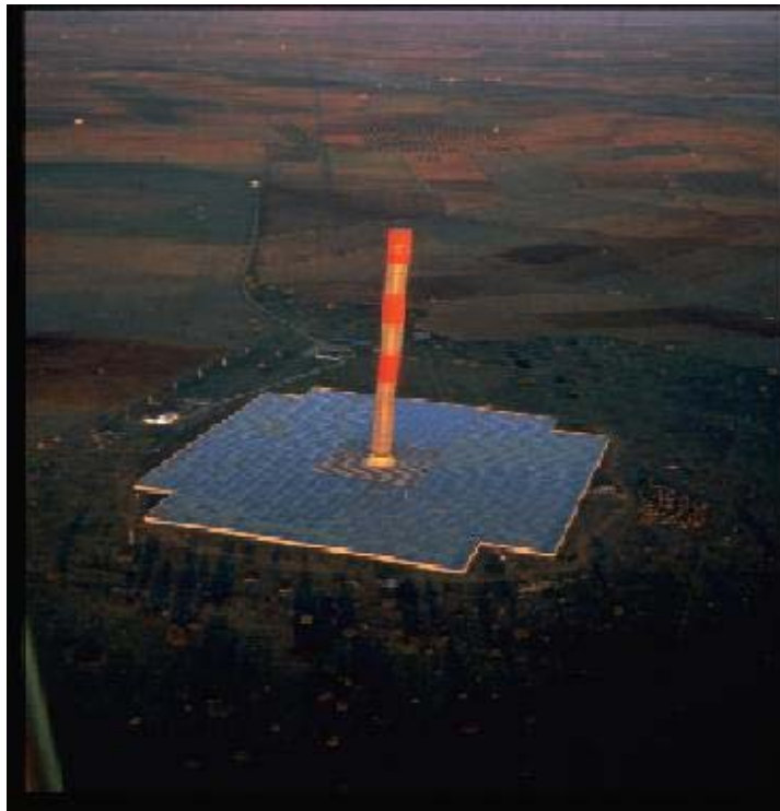
“Proof-of-technology” demonstration facility in Manzanares, Spain.
