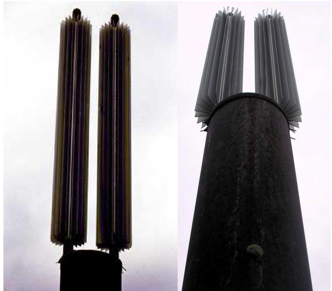
The heat pipes used to prevent permafrost melting and cool the trans Alaska oil pipeline are **12 m long**. Much longer thermosyphons have been proposed for the extraction of geothermal energy.
